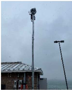
Addition of Second Accipiter® Multi-device Steerable Platform with High Powered Acoustic Hailing Device and Thermal Camera
