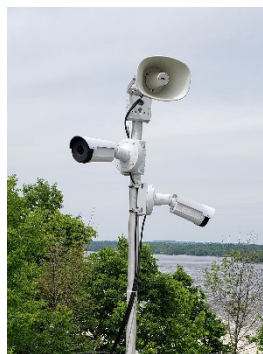
Axis 1942-E Thermal Imaging Cameras with Video Analytics Software and Axis C3003-E PA Horn
